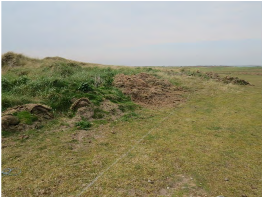
Large former waste and spoil heap back of driving range
