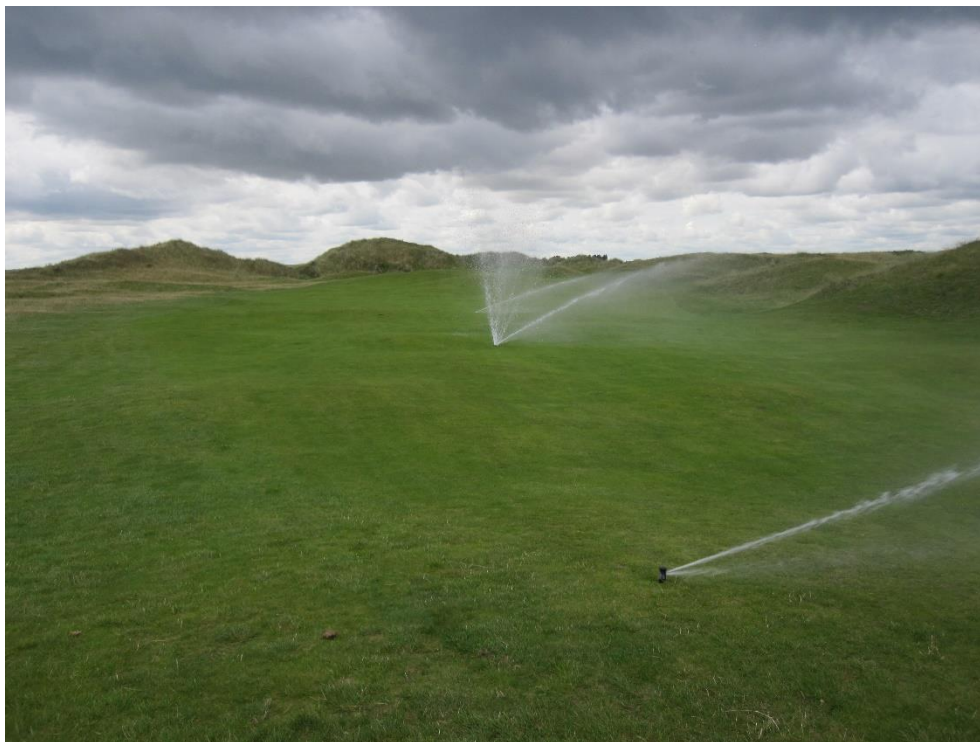
16 – Typical fairway irrigation – Note; single row and wind disturbance
