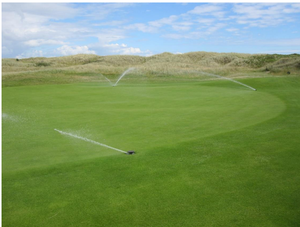
11 – Typical green irrigation – poor pressure and coverage
