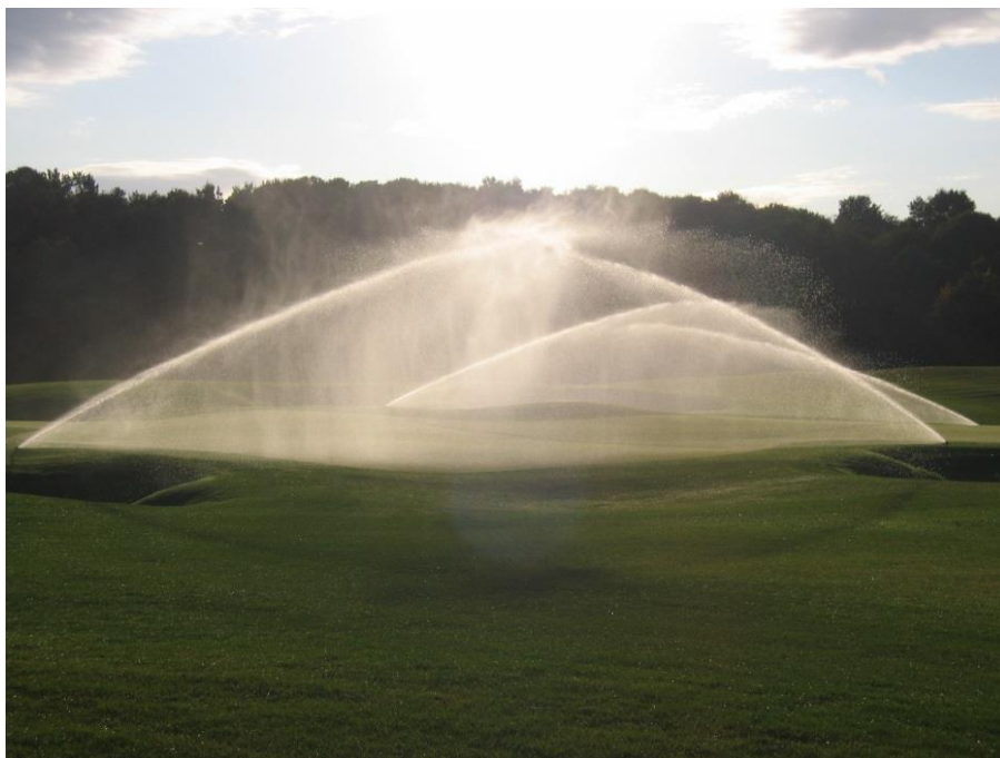
18 – Modern Valve-In Head Sprinklers in Operation [example photograph] – note good curtain of water and coverage [low angle nozzle shown for windy conditions]
