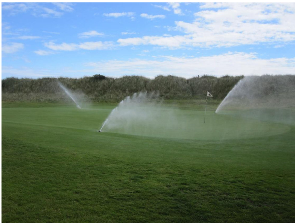
12 – Typical green irrigation – improved pressure, coverage still poor
