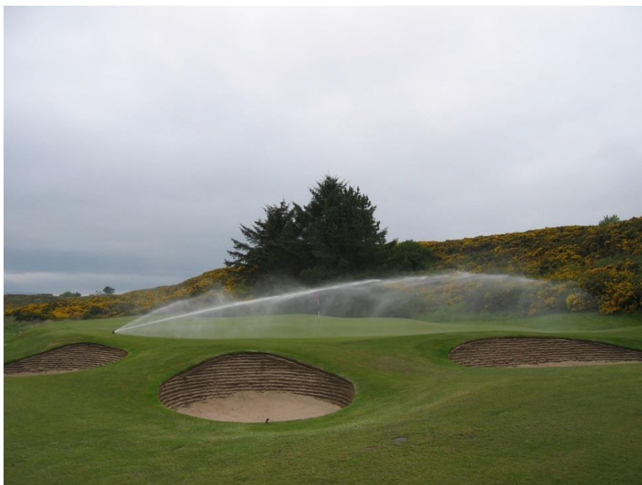
18 – Modern Valve-In Head Sprinklers in Operation [example photograph] – note good curtain of water and coverage [low angle nozzle shown for windy conditions]
